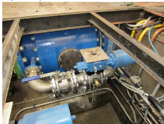
Valves under functional test in a powerplant
